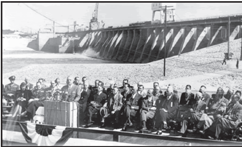
Kentucky Dam dedication, 1944; Photo courtesy of TVA files
